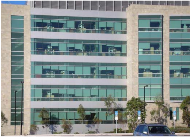
Fig. 1: Range of blind deployments at a campus building. (photo: Craig F. Johnson)
